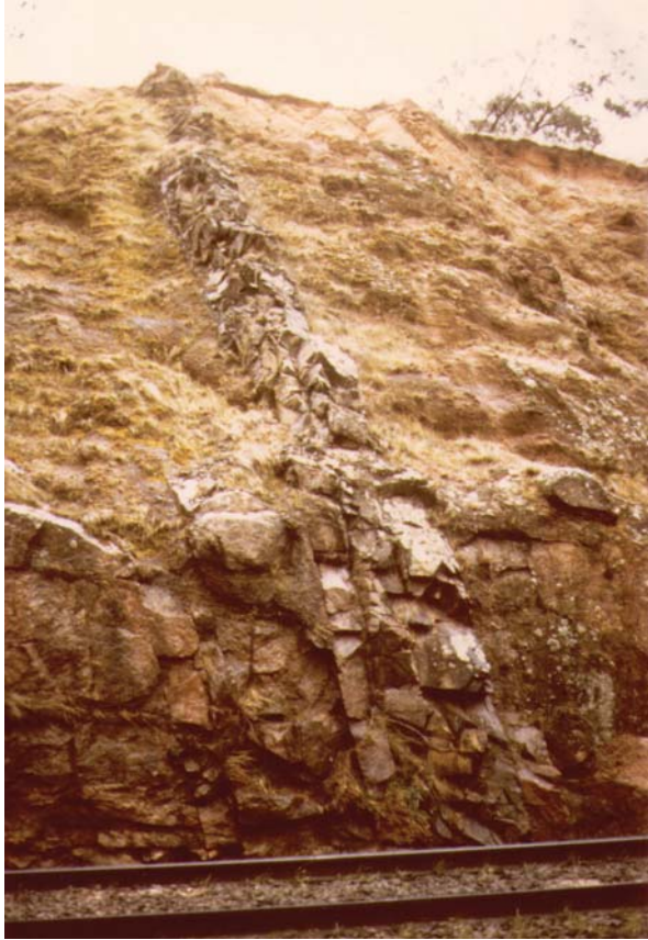
Fig. 12. A basaltic (basic) dike cutting across the Bathurst granite in a railroad cut at grid reference 948587 in Fig. 4 (from Snelling 1974). Notice the parallel jointing in both the dike and the granite, due to the basaltic magma having intruded along the jointing in the granite.
