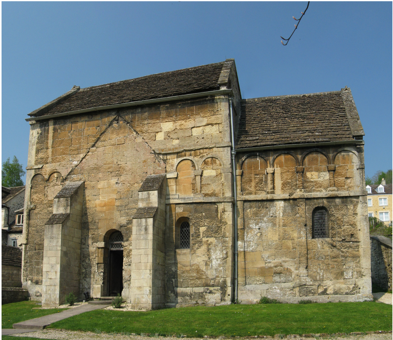
Fig. 4. St. Laurence's Church, Bradford-on-Avon, England, has two simple buttresses on each side of the entrance to support the wall. The mudbrick fortification wall of Jericho built by Hiel three thousand years ago would have had simple buttresses, perhaps similar to these. Buttresses of various styles have been used throughout history. Charles Miller, "Saxon church, Bradford on Avon," https://en.m.wikipedia.org/wiki/File:Saxon_church,_Bradford_on_Avon.jpg . CC BY 2.0.
